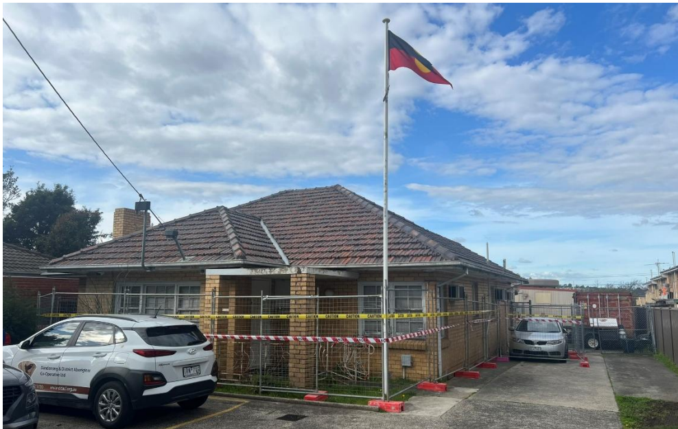
Figure 2 DDACL's main office had to be closed down in August 2024 due to asbestos
